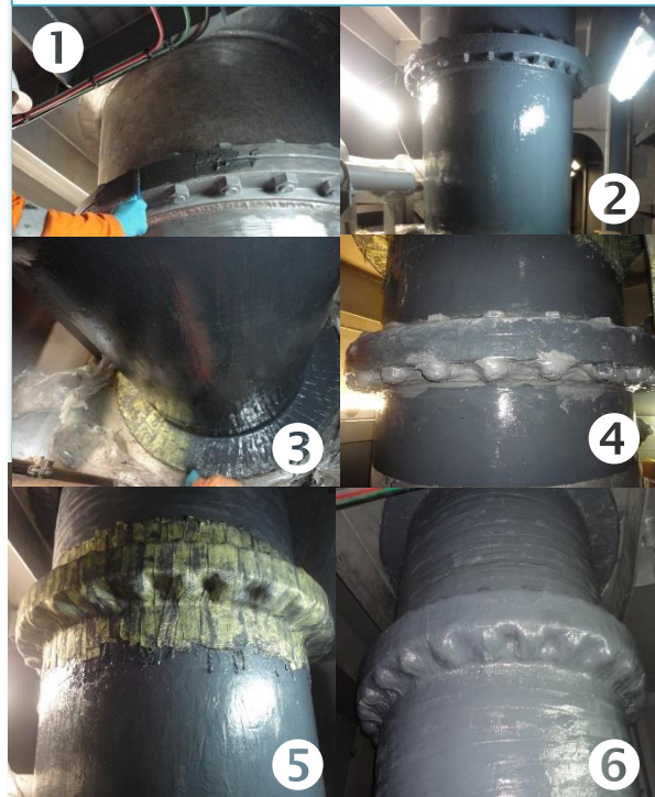
Composite repair steps
