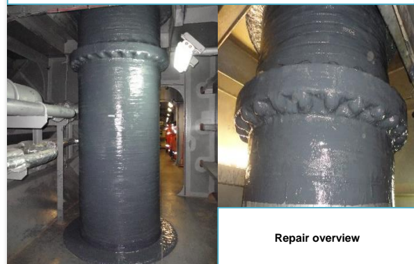
Composite repair steps
