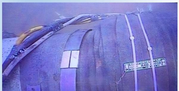
Figure 5: Subsea markers and reference plate installed
