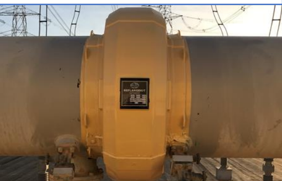
Figure 6: REFLANGEKIT® installed and recovered with protective coating
