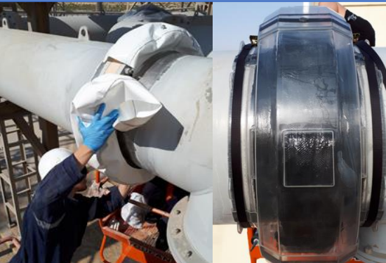
Figure 4: Soft shell installation
