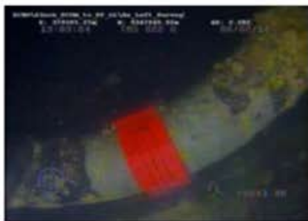
STOPKiT® successfully installed on the bend
