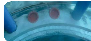
Fig. 3 Application of the composite repair material inside the groove
