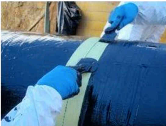
3X Engineering's composite repair
