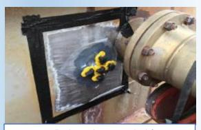
Fig. 4: Metallic plate application over the defect using magnets
