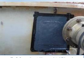
Fig. 5: Composite patching completed (5 layers)
