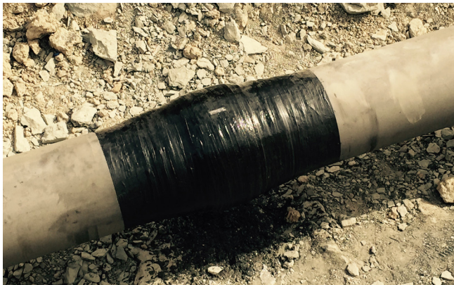
Figure 2. View of the finalised composite repair in Iran.
