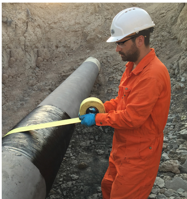
Figure 1. R4D wrapping in progress.
