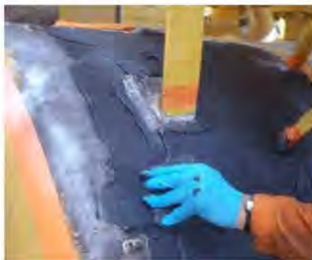
F3XS1 filler application on patch area
