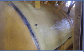
Figure 3: Composite patching finalized
