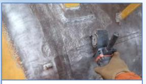
Figure 1: Surface preparation using Bristle Blaster machine
