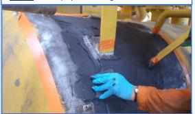
Figure 2: F3XS1 filler application on patch area
