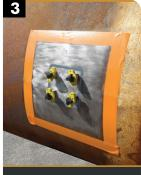
Steel plate application (with filler & magnets)
