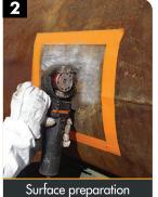
Surface preparation Sa21/2 / St3 and roughness Rz > 60 µm
