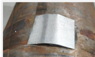
Remove ratchet belt system and galvanized steel plate
