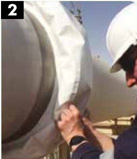
2 Leak sealing with soft cover application and valve
