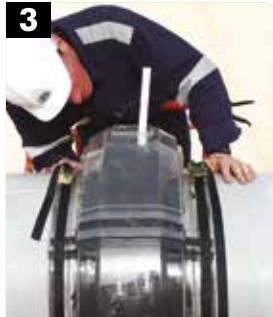
3 Hard shell installation
