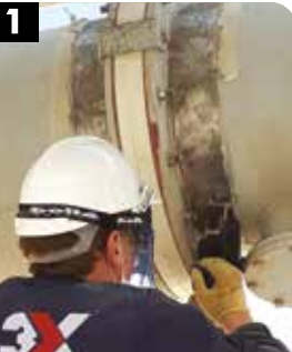
1 Surface preparation Sa2½ / St3 and roughness Rz > 60 µm
