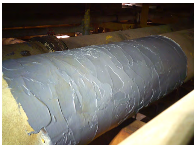
Figure 1. Case study 1: surface reconstruction with filler.
