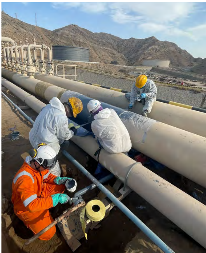
Figure 3. Case study 2: composite wrapping on progress.
